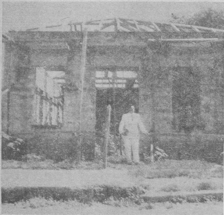
This will give you an idea how the new church building at Codajas is coming along. This is built out of tile brick and will have a tile roof. The walls will be plastered and painted both inside and out. Pastor Miguel Ibern on standing in front of building.
