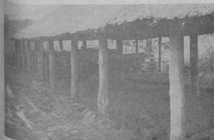
This is the drying shed. The bricks are put here for several weeks before being put into the furnace or kiln.
