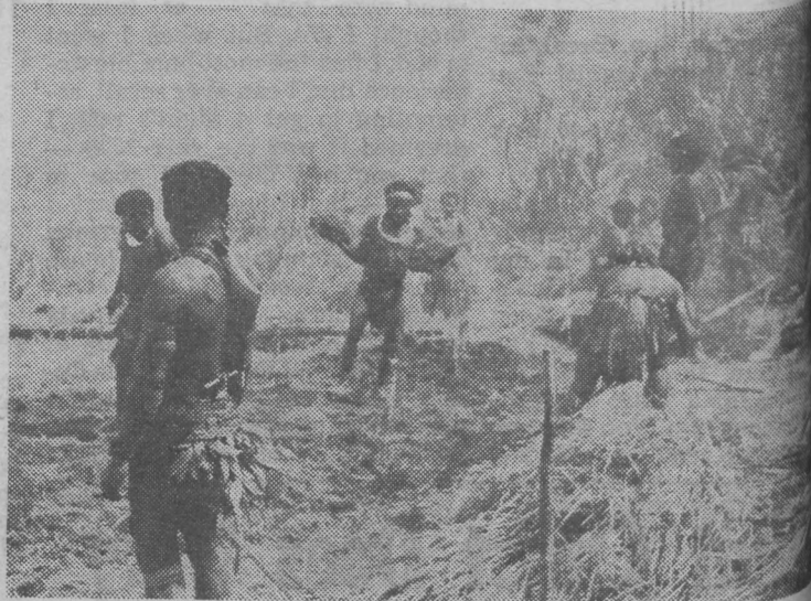
In this picture the natives are clearing the ground for the building site. Cane, brush, bamboo, vines, grass, and general jungle growth had to be removed before we could begin.
