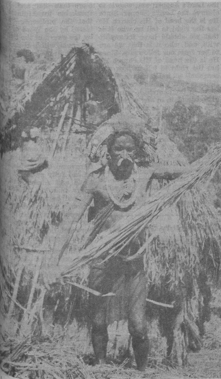
In this picture the roof is just about completed and the gable end is being covered in a similar manner. Note the crude ladder. This old man is preparing a bundle of grass to throw up to the workers.
