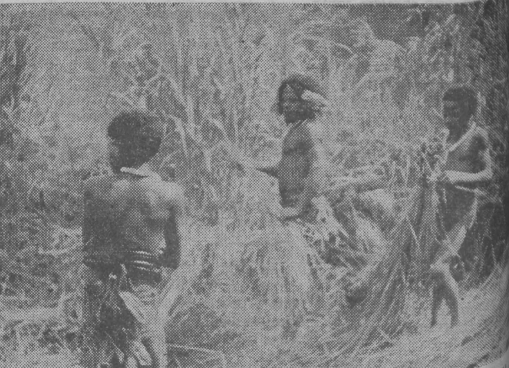
In this picture some are cutting and tying into small bundles the long grass that is used for the roof. (Continued on next page)
