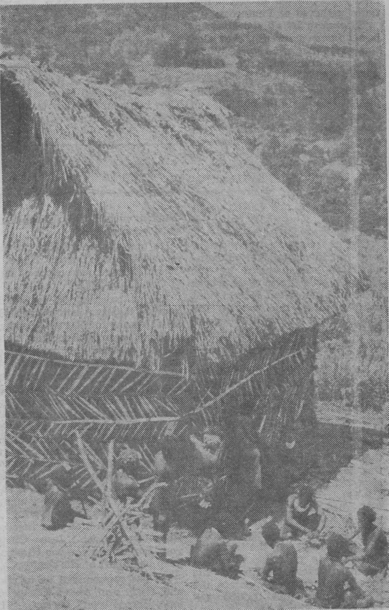
Here the house is near completion. They are working on the door. The door was made of woven material made from cane.
