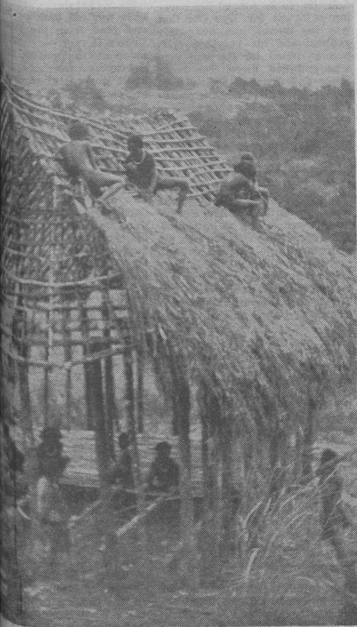
Here the grass is being applied to the roof
