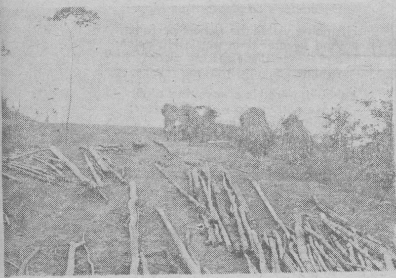
First of all the material, (most of it) is brought to the site where the building is to go up. In this picture can be seen poles and small trees scattered about the ground, also the women folk help in the building by bringing some of the material. Here the women are bringing large loads of grass for the roof and the gable ends.
