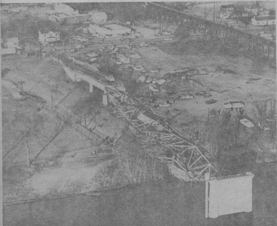
This photo was made from the West Virginia side of the river, looking toward the State of Ohio, and shows the twisted wreckage of the span of the Silver Bridge after it fell. When this portion of the ramp fell, many cars were crushed beneath it.
