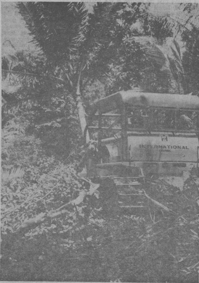
Pushing over giant trees with bulldozer to clear way for a road through the jungles of Bougainville.
