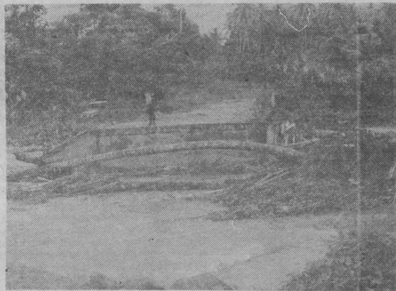
(3) Here shows another place where only the abutment was left of one bridge. Coconut trees and other debris can be seen. At the far left of the picture is a Toyota 4-wheel drive vehicle waiting for the floodwaters to go down so it can go across. These vehicles are very rugged and, except where the water is so deep and/or swift that it would turn the vehicle over, they can go most anywhere.
